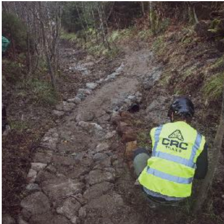
A section of hand-built trail under construction
